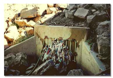
**Photograph SSC-1.** Storm drain cleaning may help to remove pollutant sources and helps to maintain the capacity of the storm pipes.
